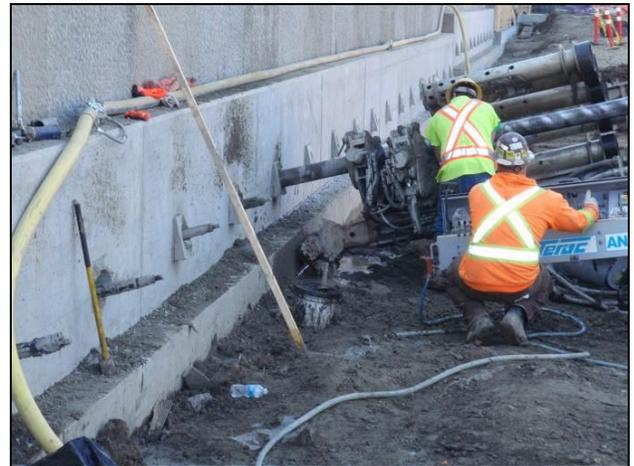
Figure 8. Drilling and soil anchor installation.
