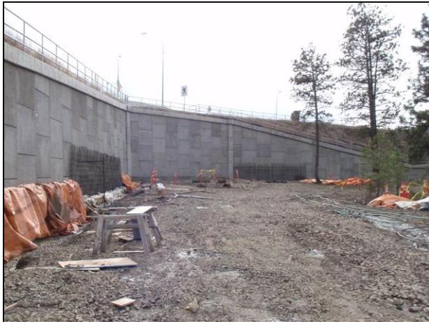
Figure 1. MSE wall prior to retrofit.
